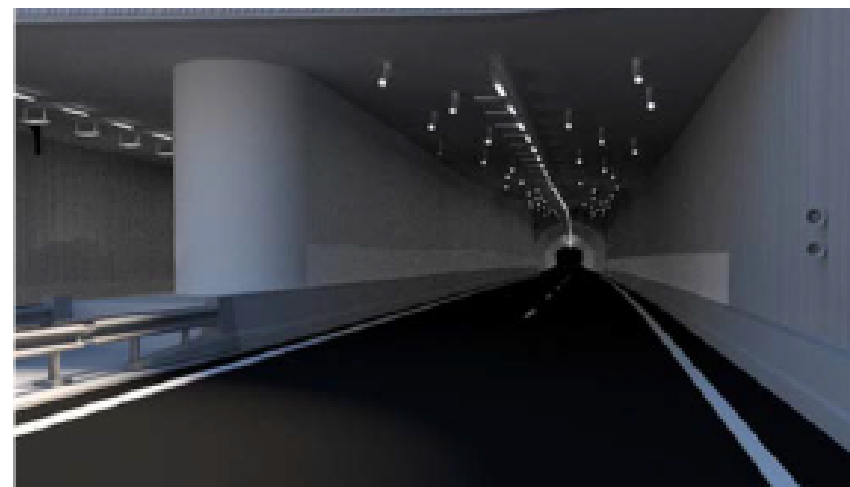
Solar optic fibre for RijnlandRoute tunnel in the Netherlands
